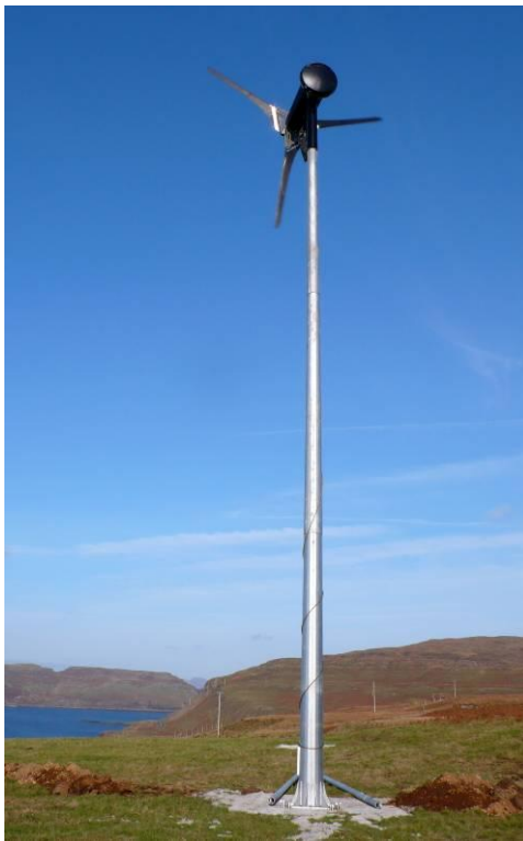
Turbine over looking Calgary Bay
