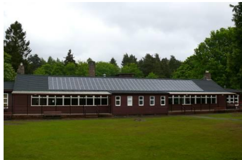
10 kWp of solar PV at Belmont Centre
