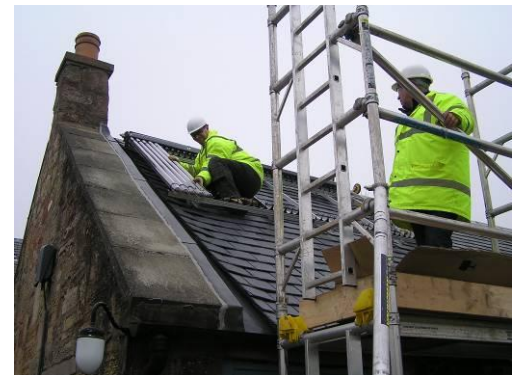
Paul installing Viessmann evacuated tubes.
