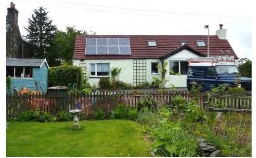
Installation near Crieff – 1.44kWp
